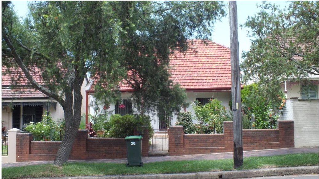
Figure 20 — View to No 20 Hastings Street showing a cottage with substantial alterations. The original timber-framed windows have been removed, opening partially infilled and aluminium windows installed. Later addition terracotta roofing tiles have been extended to incorporate the verandah. The cast-iron verandah posts and decorative filigree have been removed and glazed flooring tiles added. The original front fence has been replaced with an Inter-War facebrick fence (Source: NBRS+PARTNERS, January 2015)
