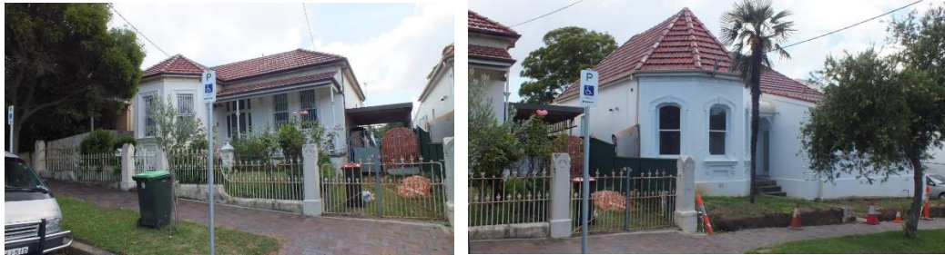
Figure 11 — View north on Hastings Street to Federation period cottages located opposite the subject group. The cottages contain original features including fence detailing with some alterations, additions and infills (Source: NBRSPARTNERS, January 2015)
