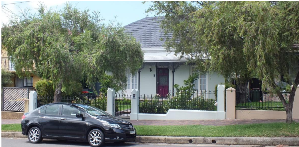
Figure 15 — View to No 16 Hastings Street showing the bullnose verandah roof in corrugated metal and the original fence elements. The original windows have been replaced with timber-framed French doors. The original slate roof has been replaced with grey terracotta tiles (Source: NBRSPARTNERS, January 2015)
