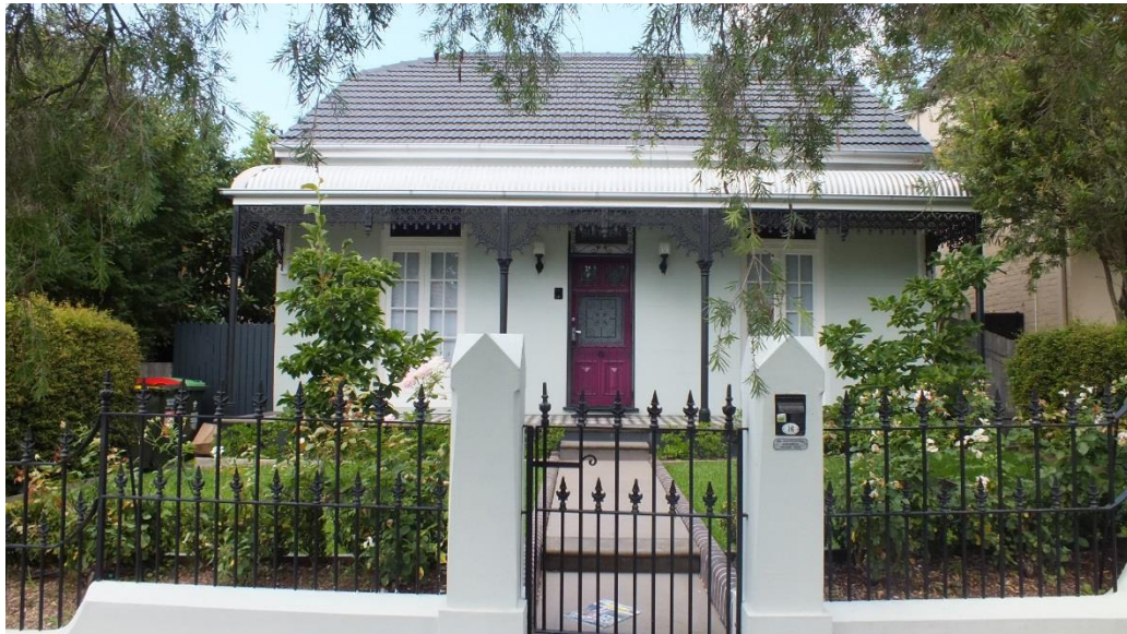
Figure 17 — View to No 16 Hastings Street showing the timber-framed front door with fanlight over, French doors with fanlights over appear to replace the original full-height timber-framed sash windows to rooms either side of the central hall (Source: NBRSPARTNERS, January 2015)
