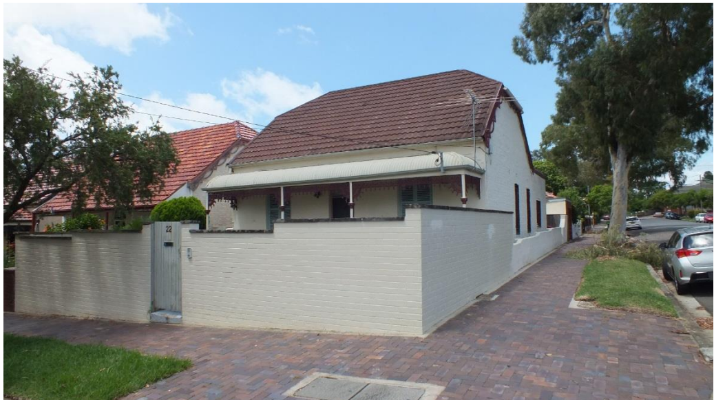
Figure 21 — View to No 22 Hastings Street, showing the cottage located on the corner of Anderton Street. The closed shutters prevent inspection to determine whether original timber-framed windows are extant. The bull-nosed verandah roof has been retained, original cast-iron verandah posts and decorative filigree are retained. The tall late-twentieth century painted face brick fence obscures views to the property (Source: NBRS+PARTNERS, January 2015)
