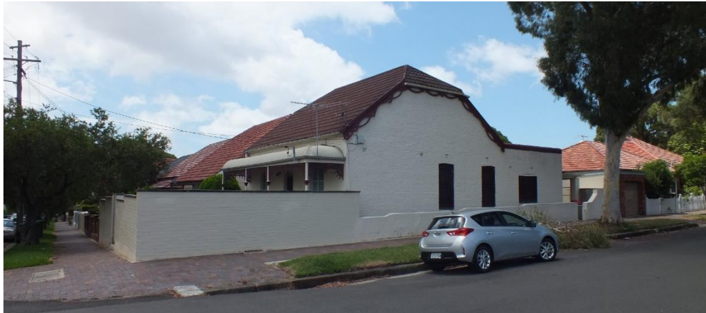
Figure 22 — View to No 22 Hastings Street from Anderton Street showing the profile of the half-hipped roof with decorative timber bargeboard (Source: NBRSPARTNERS, January 2015)
