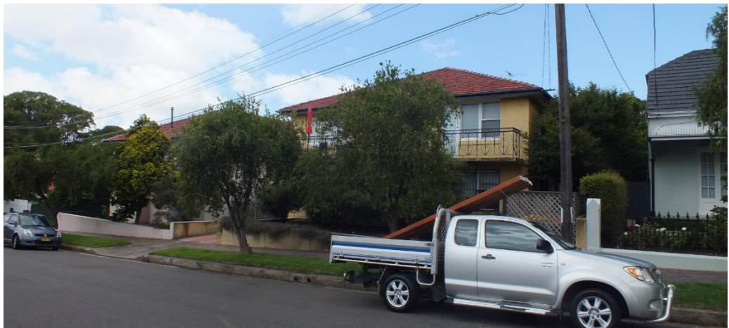
Figure 12 — View to Hastings Street, southeast of the subject group, shows a late-twentieth century, two-storey residence constructed on the site adjoining No 16 Hastings Street (Source: NBRSPARTNERS, January 2015)
