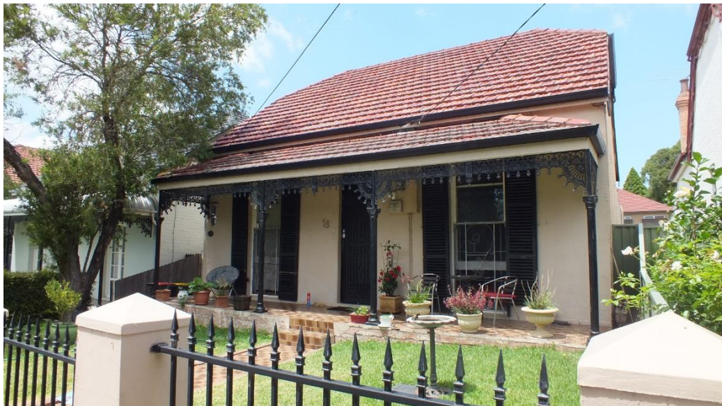
Figure 19 — View to No 18 Hastings Street. The verandah flooring has been altered with the introduction of glazed flooring tiles (Source: NBRS+PARTNERS, January 2015)
